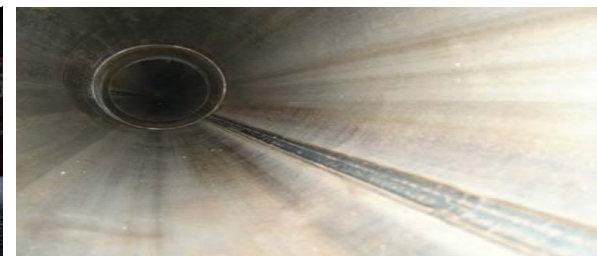
After pig cleaning
