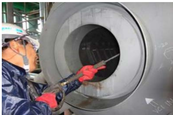
Steam Drum Jet Cleaning
