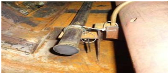
Steam Drum Inside Test Piece Install
