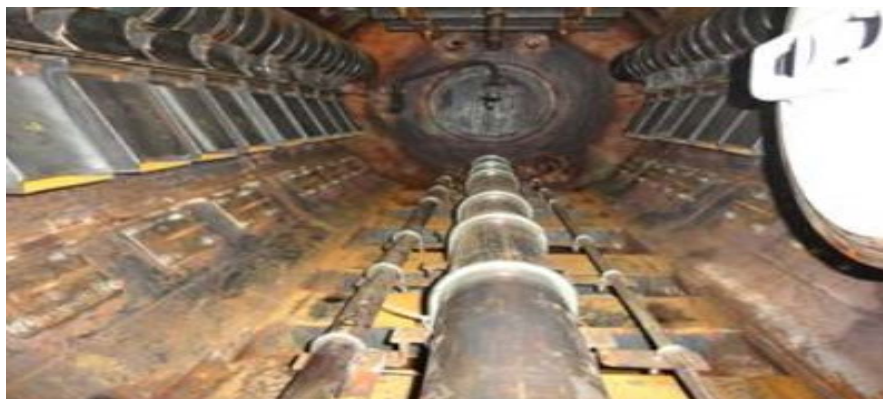
Before chemical cleaning Steam Drum
