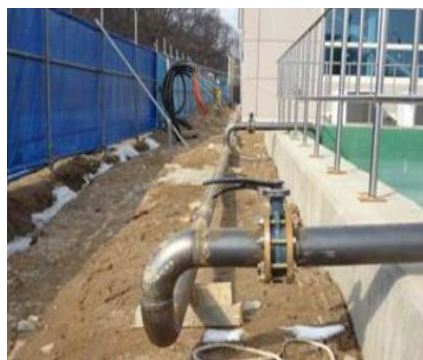
Temporary Piping Waste Water Transfer Line
