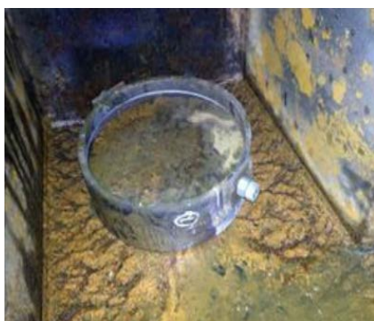
Downcomers Orifice plate install
