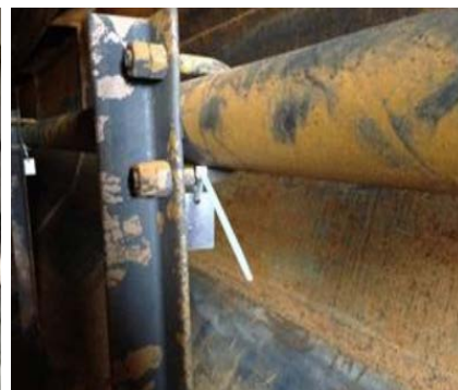
Steam Drum Inside Test Piece Install
