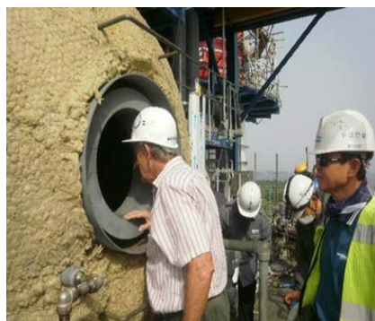
Chemical cleaning after inspection
