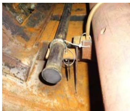
Steam Drum Inside Test Piece Install
