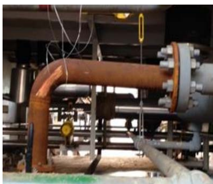
Temporary Piping HP Evaporator Supply Line
