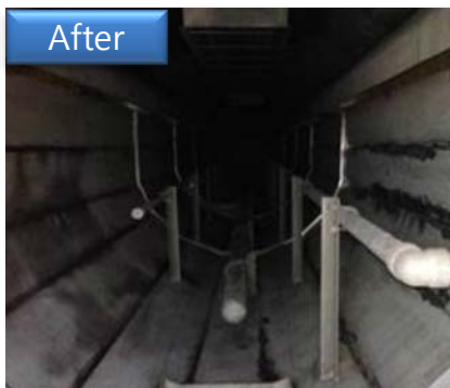
After chemical cleaning Steam Drum
