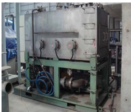
POSCO-Vietnam Cold Rolling Mill Plant
