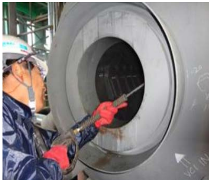
Steam Drum Jet Cleaning
