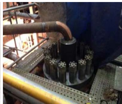
Temporary Piping HP Main Steam Return Line
