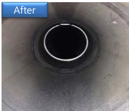
After chemical cleaning Condensate Line
