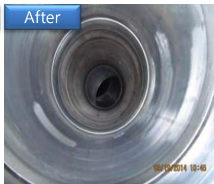
After chemical cleaning Adsorbent chamber bed line
